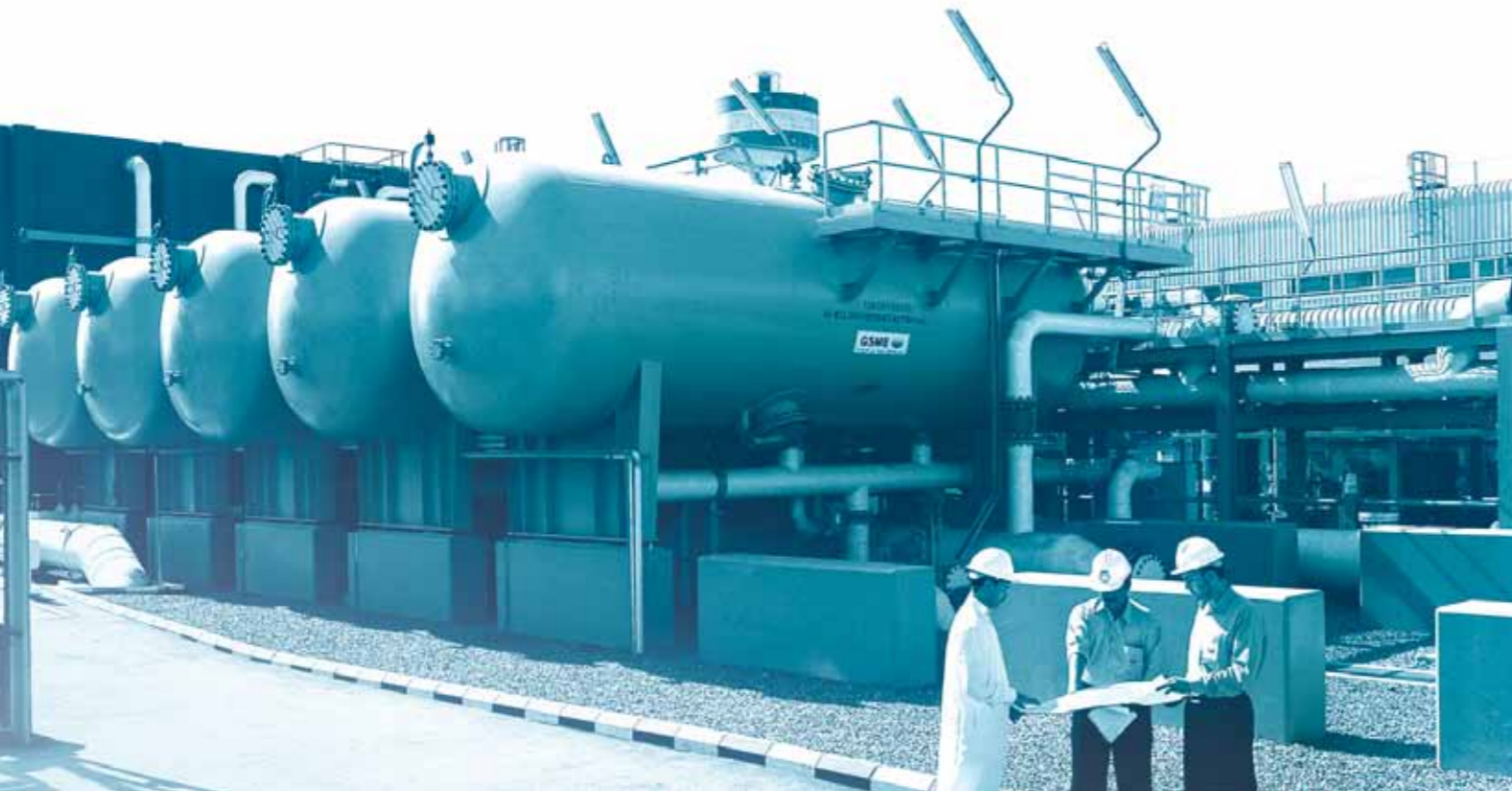
50,000 m 3 /day seawater membrane filtration system
